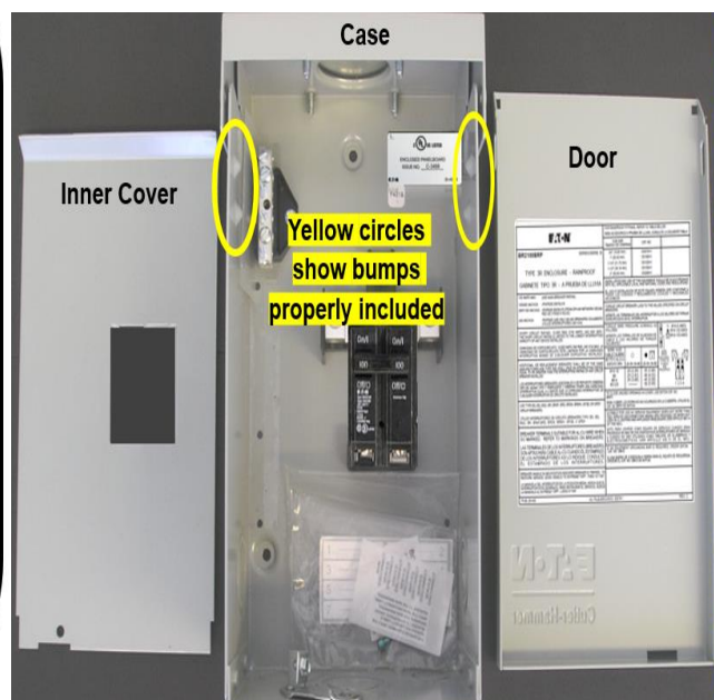
Figure 4. Identification of bumps feature location inside case
